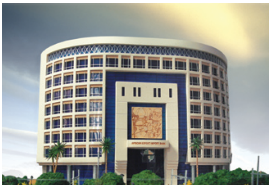
Model of AFREXIMBANK Headquarters Building (under construction)
